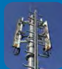
Broadband base station in Stuttgart
